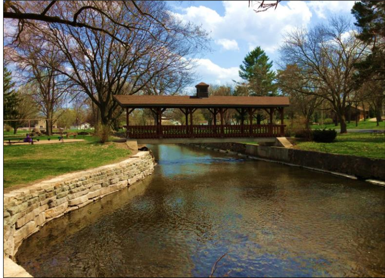
FIGURE 6B: BRIDGE OVER ALLEN CREEK AT LAKE LEOTA PARK.
